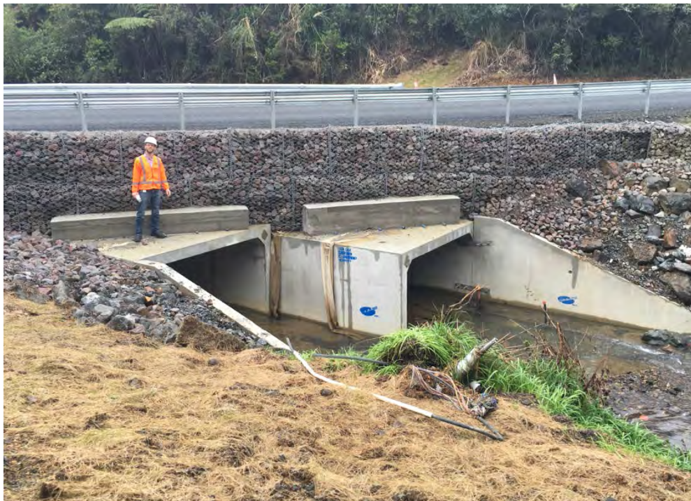
Picture 1: Completed twin culvert replacement at Rotowaro Road
