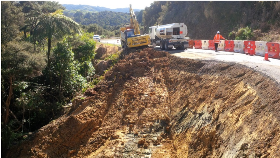
Picture 1: Slip repair at Ohautira Road
