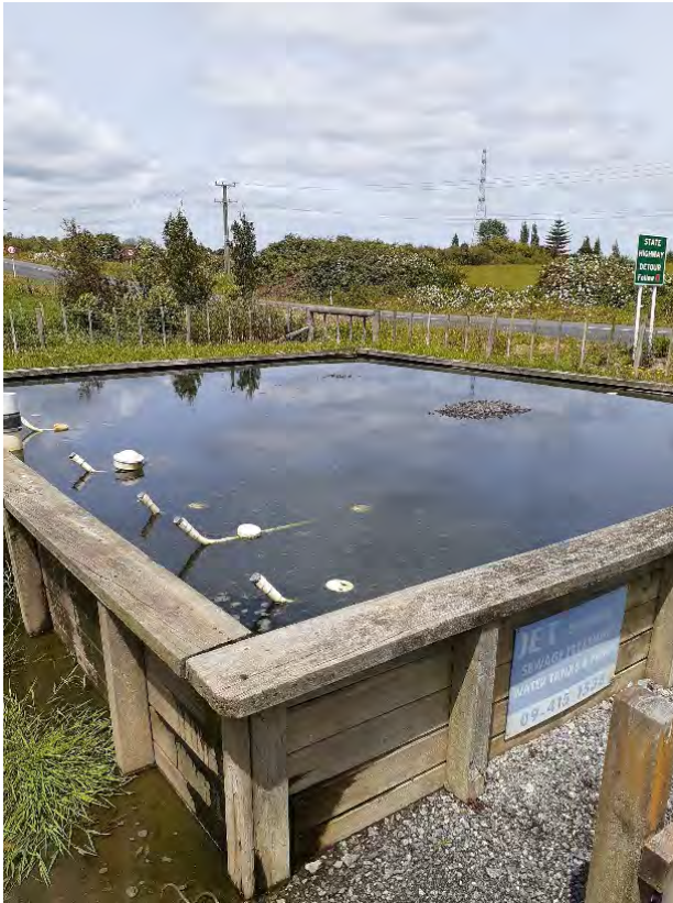
Maramarua WWTP prior to media replacement
