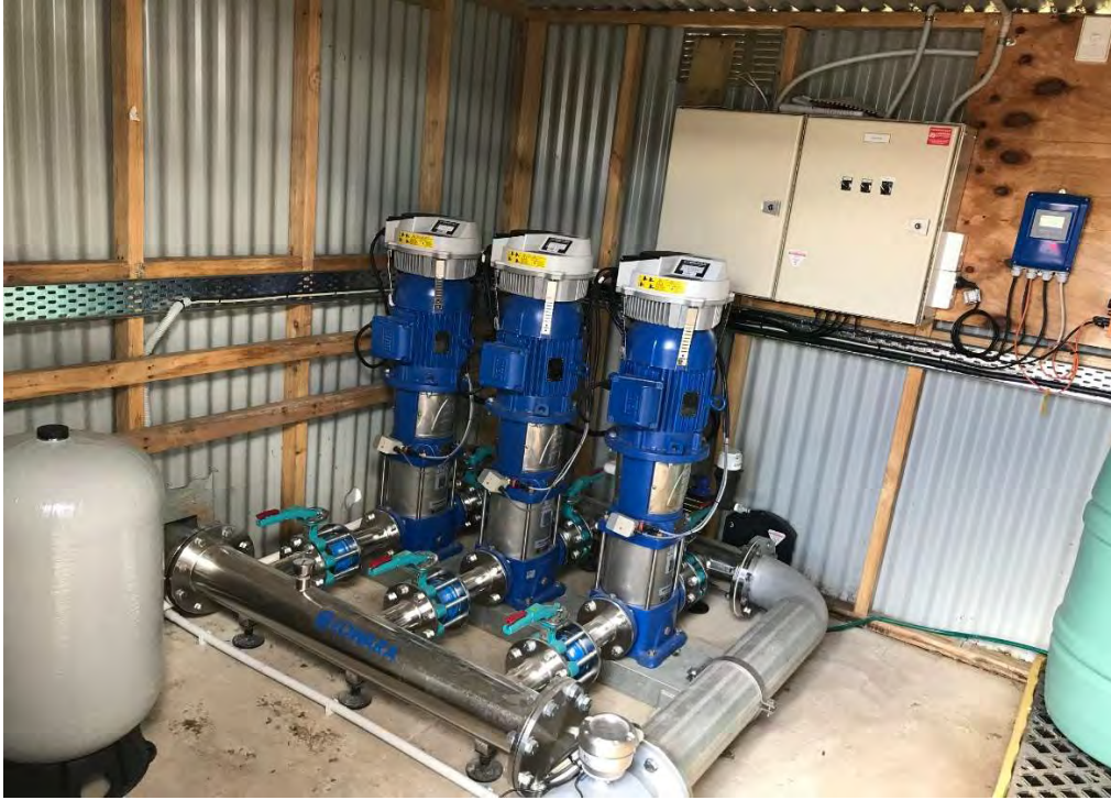
Puketaha Booster PS after the upgrade works had been completed.
