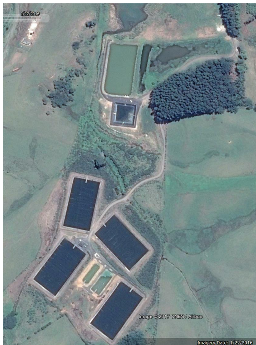
Aerial view of site
