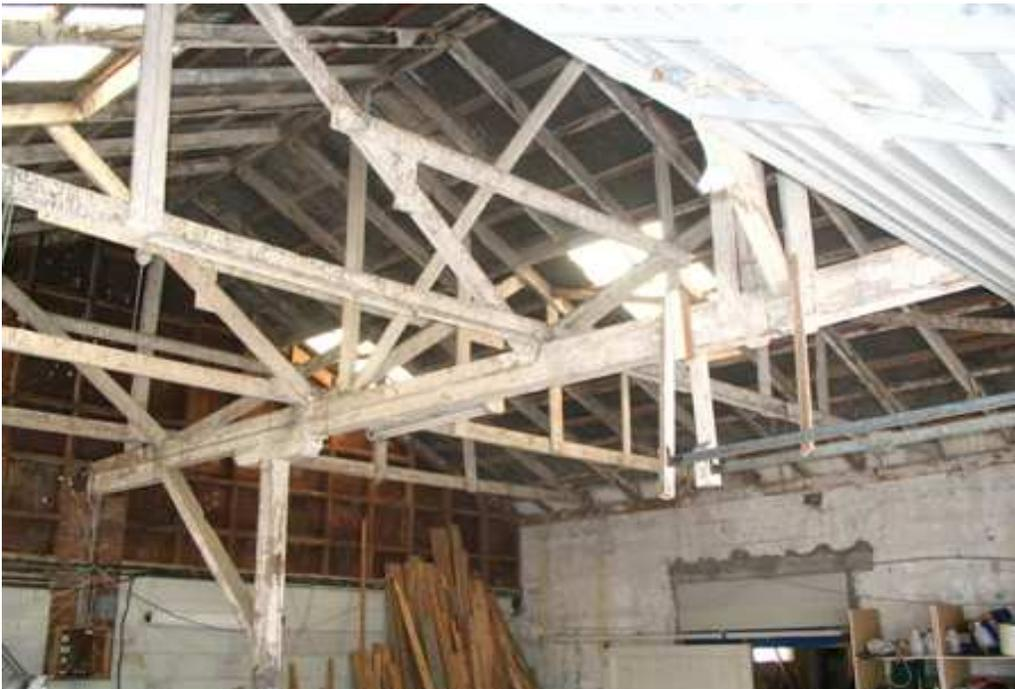
**Huge sandwich style beams bolted together make up the truss work inside the building to the immediate left of the original factory.**
