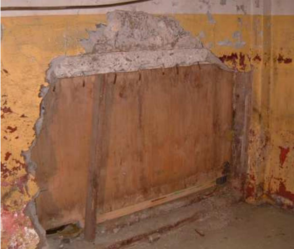
**Hole where front end loader has been driven into the wall**
