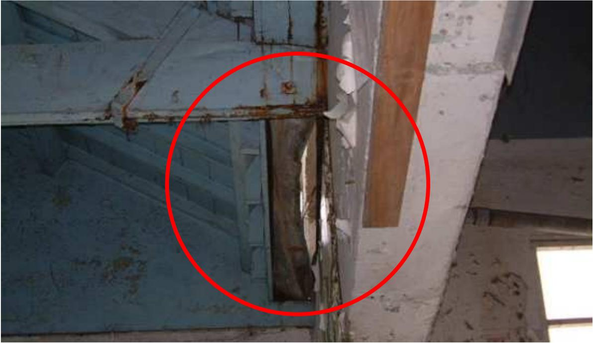
**Collapsed tin gutter.**
